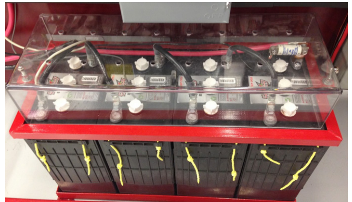
Figure 14. A bank of 6 volt batteries connected in a series string. Batteries store DC energy.
