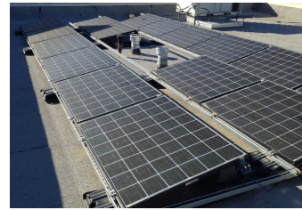
Figure 4. Modules mounted together on racks and wired together to create series strings. Arrays can be pole-mounted (left), ground-mounted (right). Roof-top arrays (below) can be mounted using flat-roof racking, and pitched-roof mounting systems
