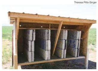
**Figure 7.17** A simple shelter design using dimensional lumber, plywood, and corrugated metal.
