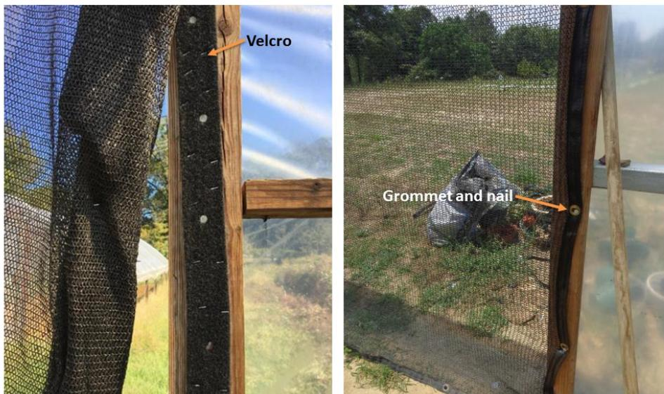
Fig. 5. On-farm methods for securing shade cloth to the end walls of the high tunnels.
