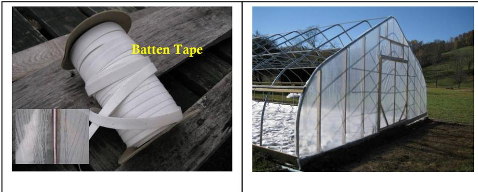
**Figure 14.** Batten tape is used to secure the plastic to the end wall frame.
