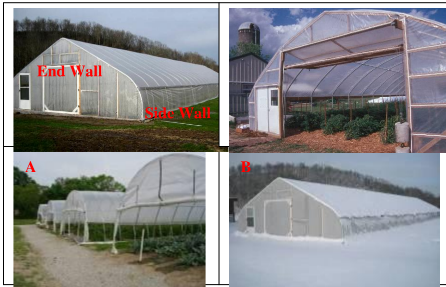
Figure 3. Quonset- (A) and Gothic- (B) shaped high tunnels.
