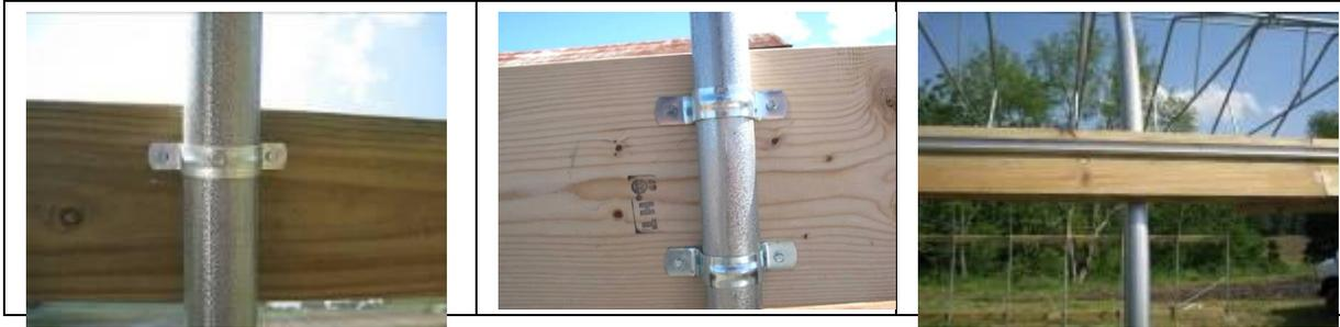
**Figure 9.** Pipe straps are used to secure the baseboards and hipboards to the high tunnel frame. Aluminum channel lock is used to secure the plastic to the frame.
