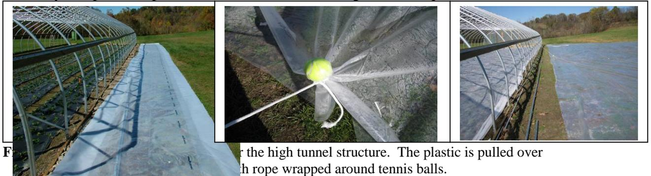
**Figure 11.** Plastic is pulled over the high tunnel structure. The plastic is pulled over with rope wrapped around tennis balls.
