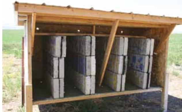
**Figure 7.17** A simple shelter design using dimensional lumber, plywood, and corrugated metal.
