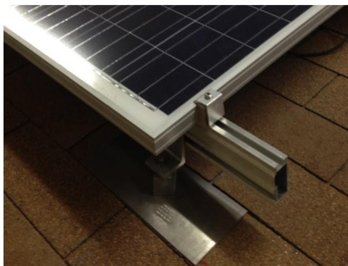
Figure 2. A roof-mount system for an asphalt shingle roof includes aluminum flashing and mounting materials such as L-feet, rails, and clamps to secure the modules in place.
