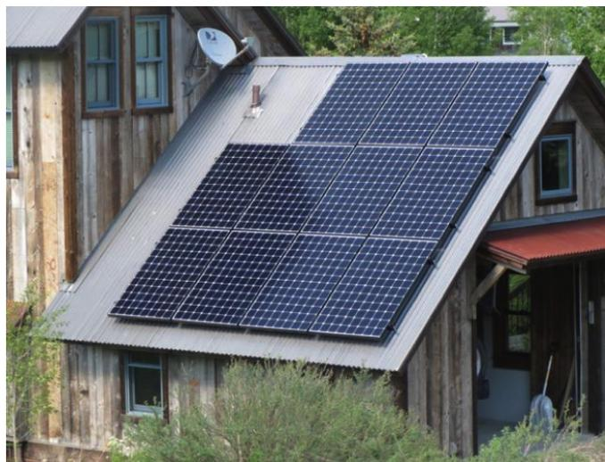
Figure 1. A roof mount array on a pitched roof. There is open roof space on all sides of the array for access. The empty space is next to the roof vent. Courtesy Nunatak Alternative Energy Solutions
