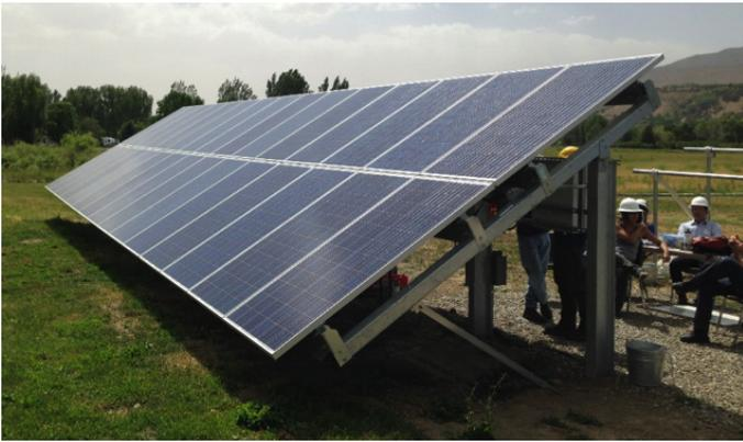
Figure 7. Solar modules arranged in two rows on a large fixed-plate ground mount system. The larger size modules require larger mounting materials to support the weight and to keep the system stable during high wind winds and at a tilt angle to allow snow loads to be easily removed.
