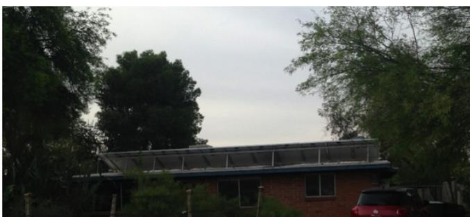
Figure 4. Tilt-up mounting systems on low slope or flat roofs are a method to set the tilt of the array to the latitude of the location to maximize the energy output of the array. Although this system is facing south, shading cast on modules from nearby trees can limit the amount of energy an array is capable of producing.
