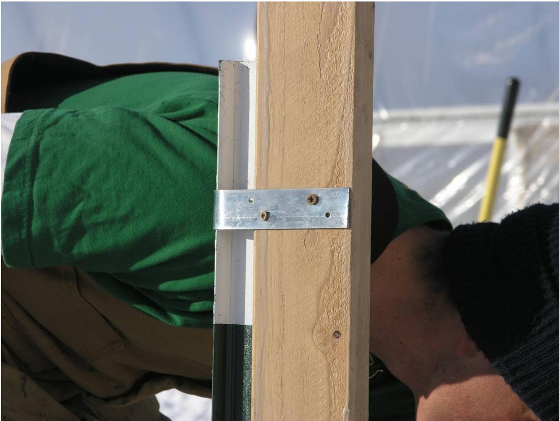
**Attatch end wall to t-posts with plumbers strapping**
