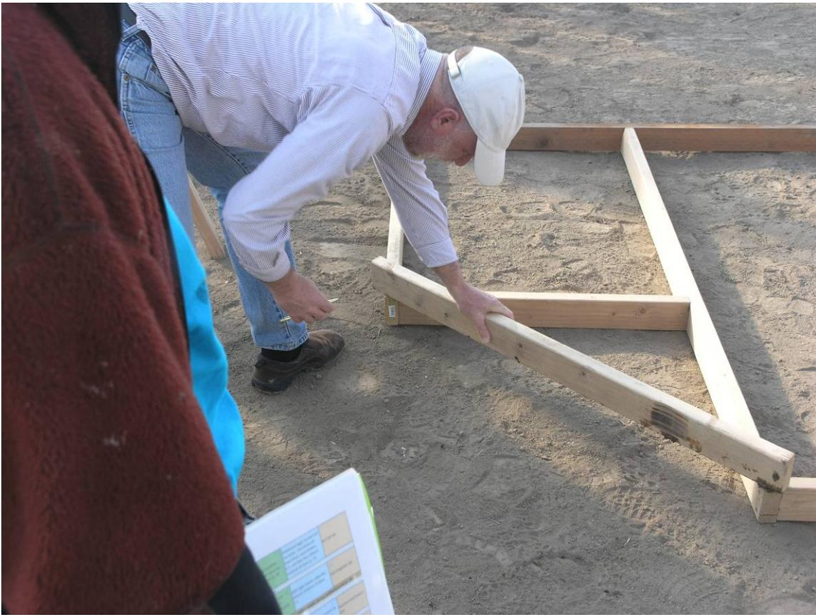
Mark cutting angles for boards "I" and "L" by laying them on top of adjacent boards
