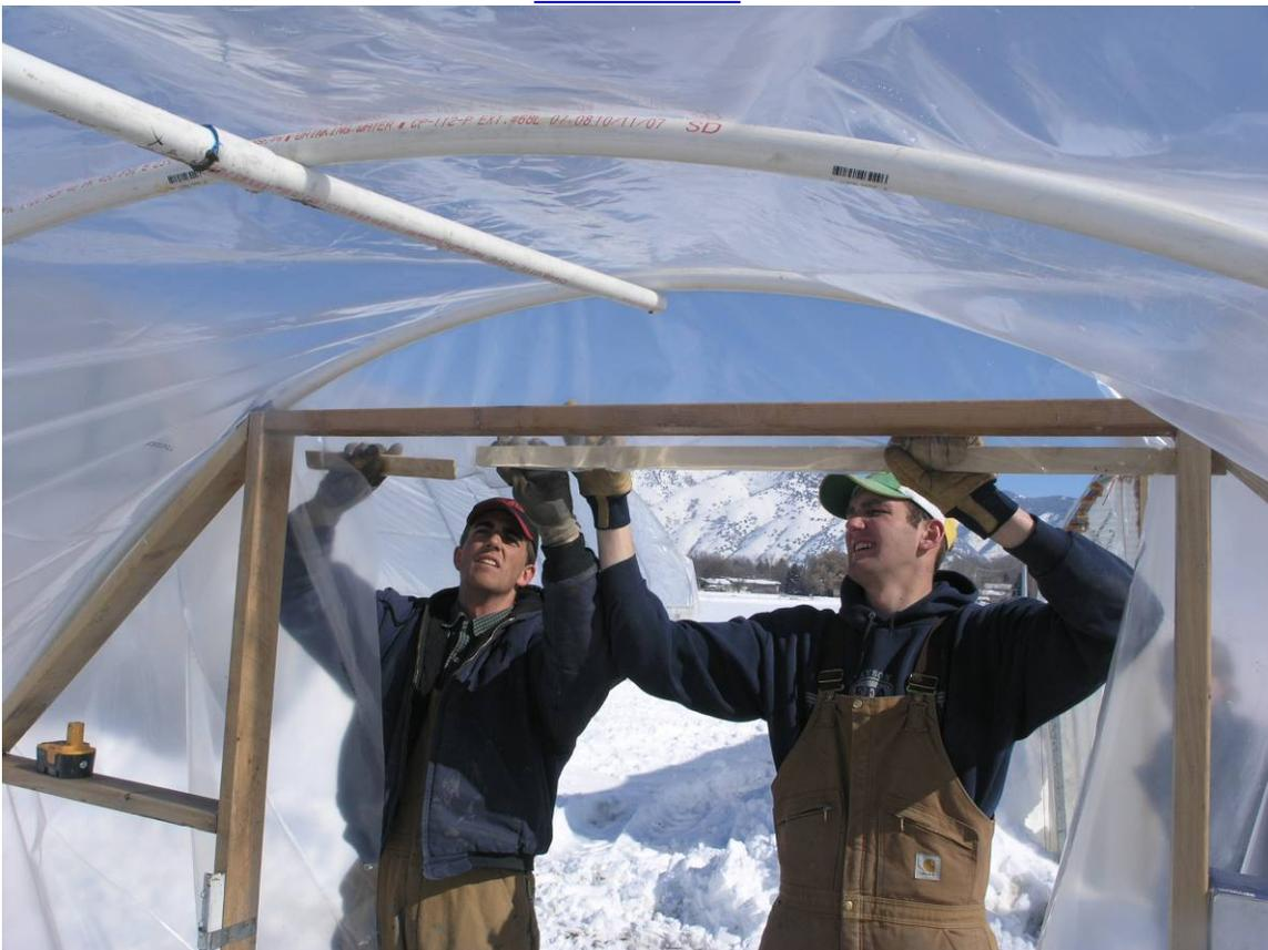
**Attach plastic to door header with lathe board**
