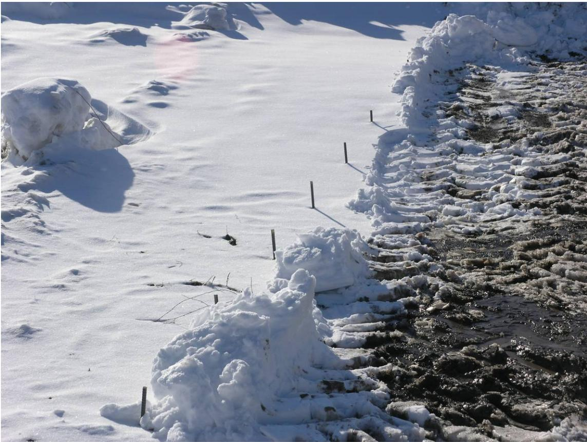
**Drive 24 inch rebar stakes 18 inches into the ground**
