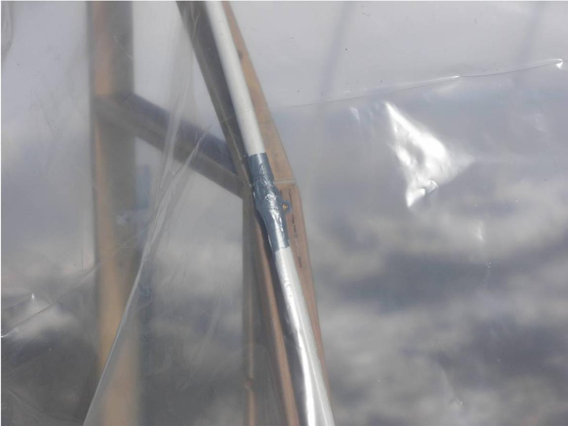
**Fasten end arches to the pre-constructed end walls with plumbers strapping. End arches should contact the end wall at the top corners of the door frame, as well as at the hip locations (shown above). Duct tape can be used to ensure that the plumbers strapping does not rip the plastic.**
