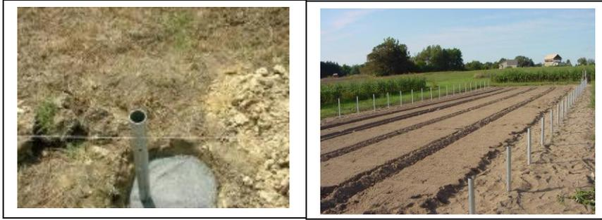
**Figure 7.** Corner posts can be set in cement to provide strength for the high tunnel structure. A leveling line is used to ensure each ground post is level. (Photo credit: A. Montri)
