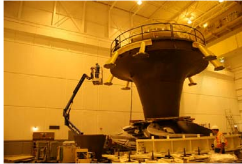
Above, workers outfit one of the turbines for Wanapum Dam. Below, tour participants inspect the new fish ladders being installed at the dam to help salmon and other fish navigate the river.
