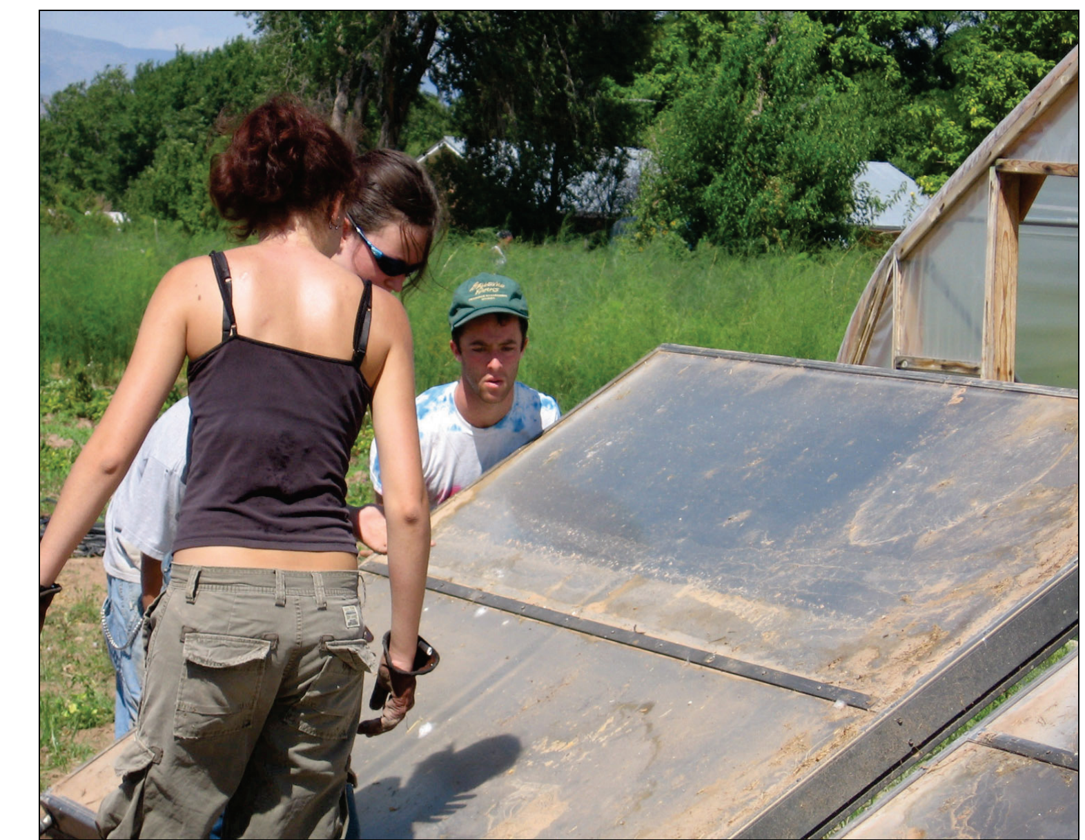
Workers help install solar panels.
