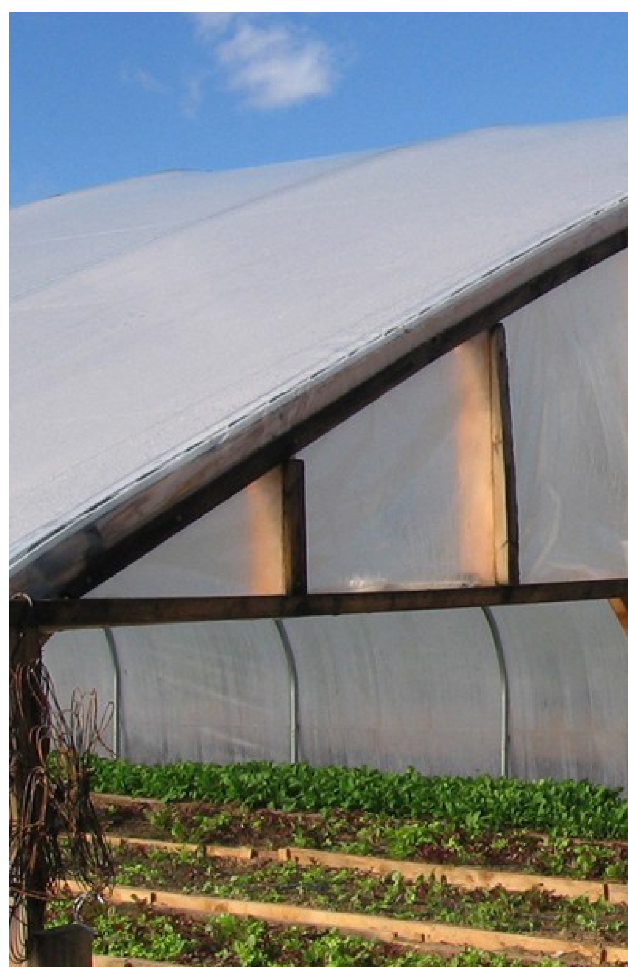
Distance education tools included an instruction DVD on building a cold-frame hoophouse.
