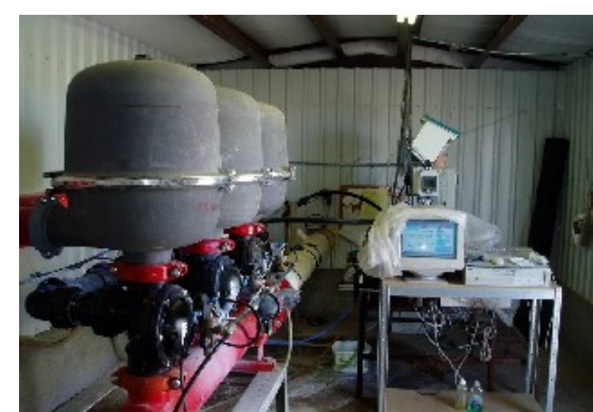
Computer controls and filters for the drip system.
