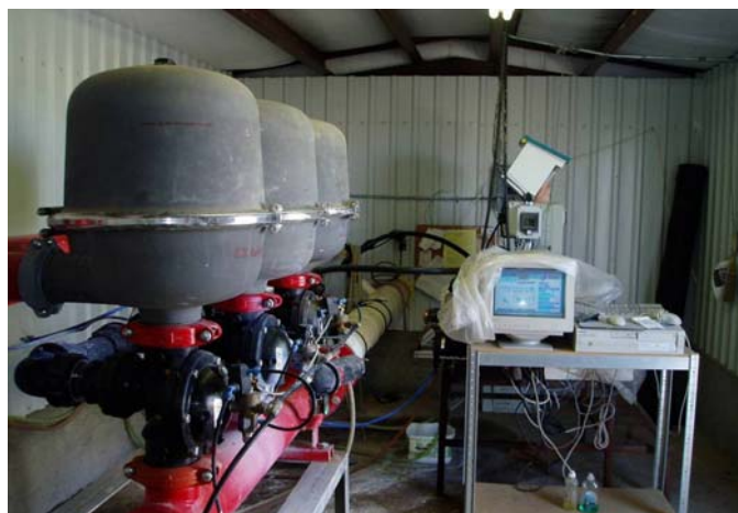
Computer controls and filters for the drip irrigation system.
