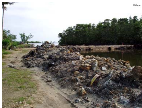
The dam, with flow gate for water exchange.
