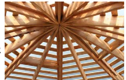
Visitor kiosk under construction.
