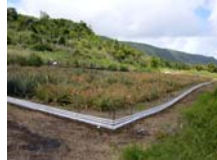
The finished electric fence stands about 14 inches high and cost less than $500 to build
