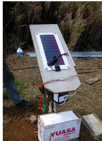
The fence was charged with a flexible solar panel
